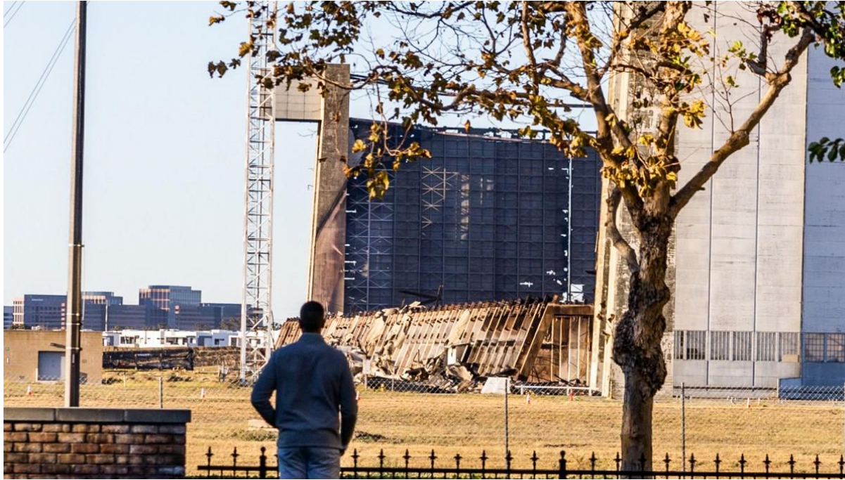
A view of the collapsed hangar from Montgomery Square Park on November Nov. 9, 2023. Credit: JULIE LEOPO, Voice of OC
